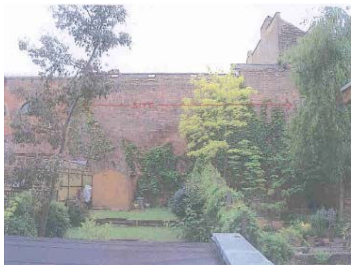
Views from Holmesdale Road
